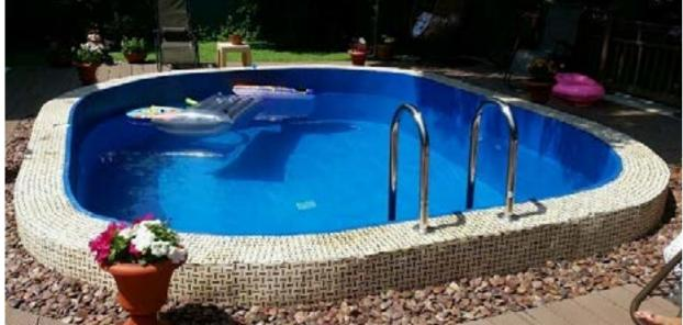
The copolymer composition is applied using a «cold» procedure; the composition is hardened by evaporating the solvent with a dry residue of at least 60%. Any color is available.
